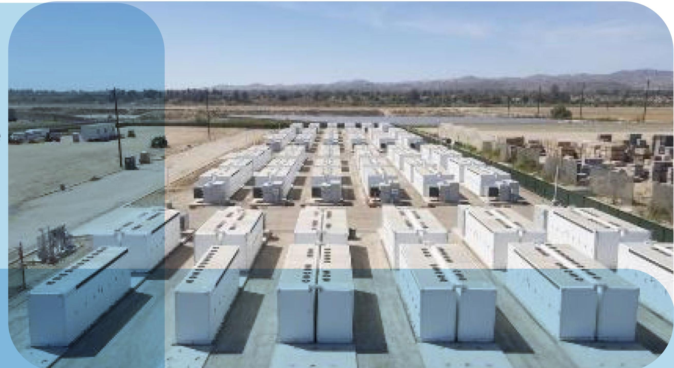
Each BESS container is equipped with a monitoring system and automatic shut off systems for enhanced safety.
